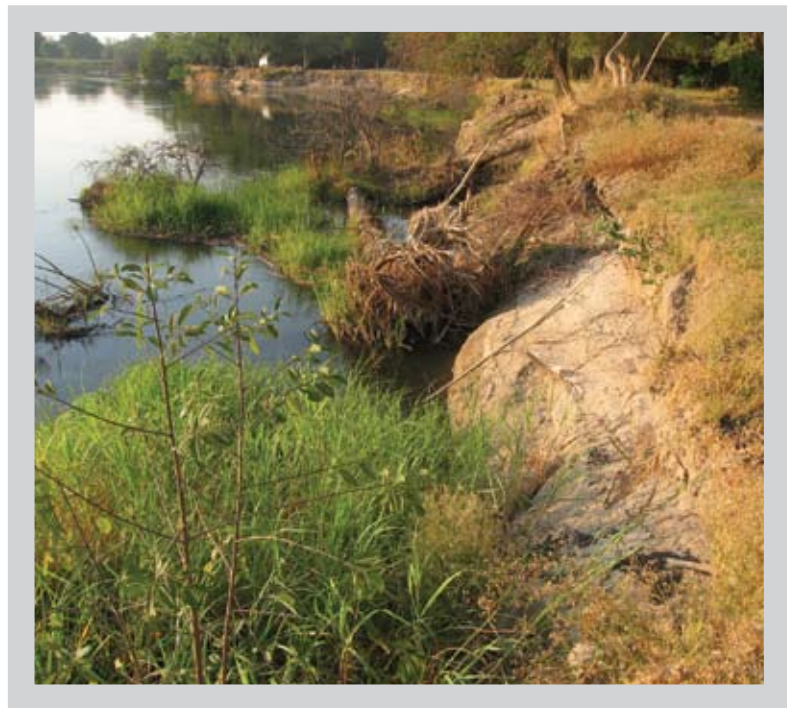
River bank erosion, Shakawe, Botswana, 2008
