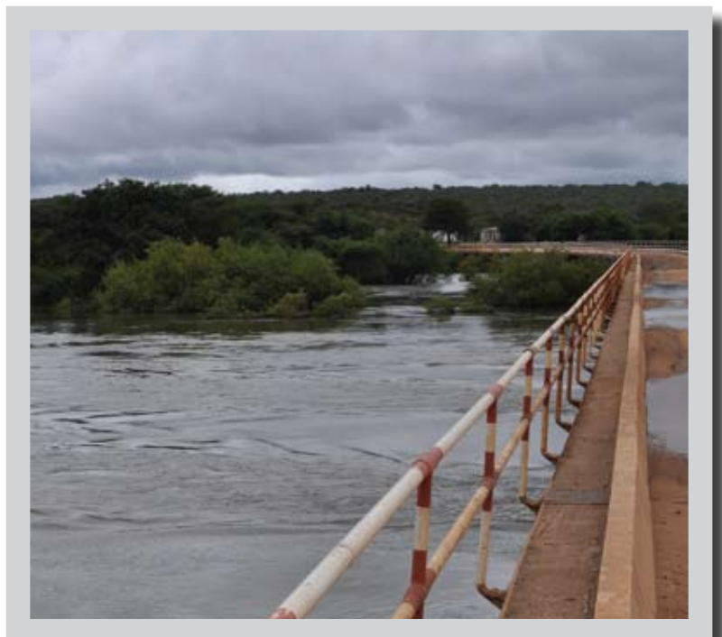
Bridge over Cubango River, Angola, 2010
