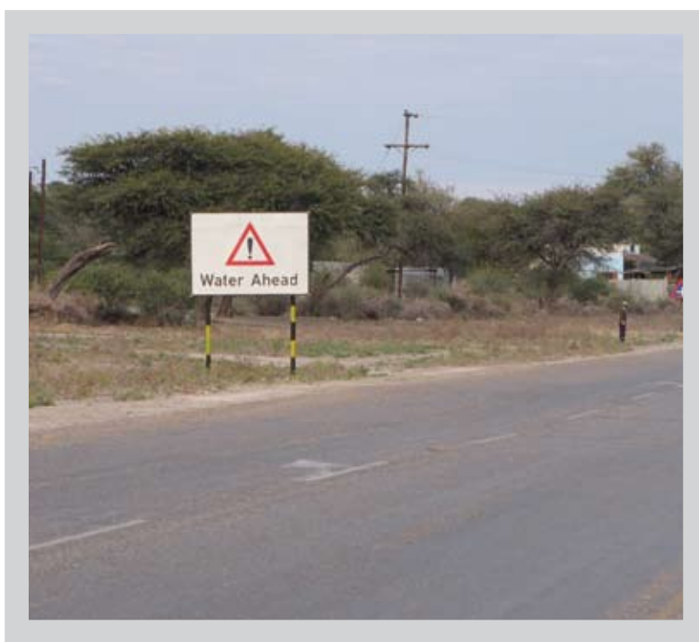
Flooding at Toteng Bridge, Botswana, July 2010
