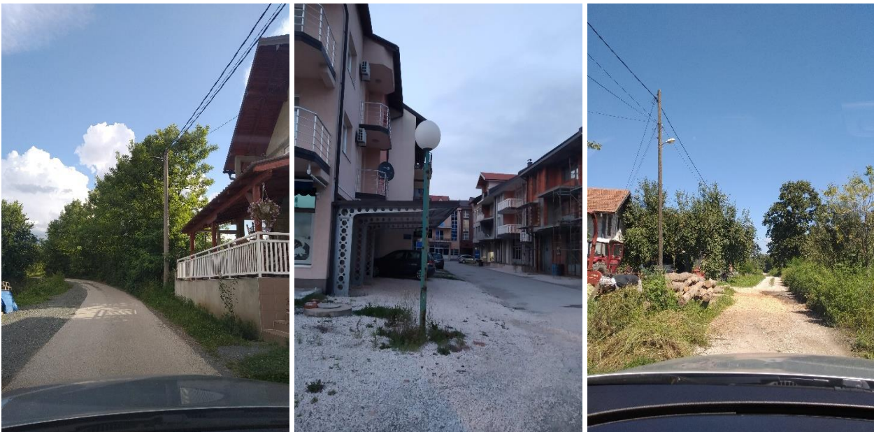
Image 27: Poles (Reinforced concrete - left, metal – centre, wooden - right)
