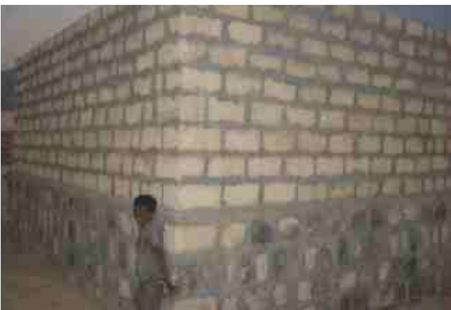
Earthquake Safe House under Construction under Indira Awas Yojana
