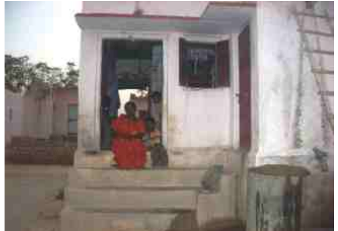
An Earthquake Resistant House under IAY
