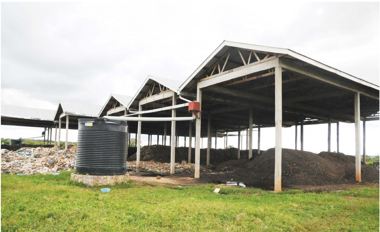
A composting plant and landfill in Aler village in Adekokwok Sub-county.
