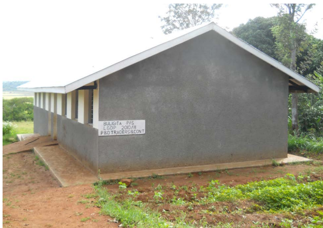
A primary school classroom block in Yumbe District
